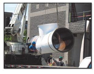
Built to ASTM 3982-08 standards for Glass Fiber Reinforced Thermosetting Resin Ducts. Our duct is built in strong light weight sections to be installed at the site. The sections are designed to minimize joints and yet ease installation and handling.
