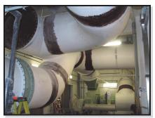
Fast on site seaming of duct allows for exact fit to valves, fans, scrubbers and vents.
